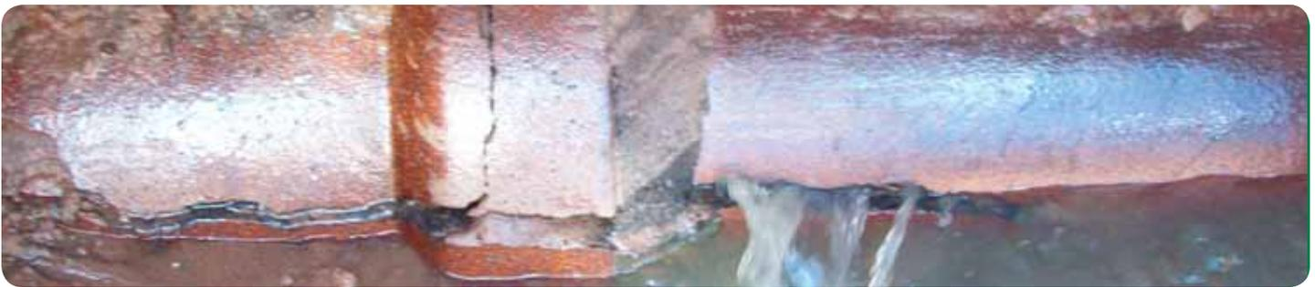
During a routine sewer line check, the PMUA discovered that an 18 inch sewer line (clay pipe), which is 80-100 years old and carries 50% of Plainfield's sewage, was severely damaged and not working properly. Designated as the Rock Avenue Interceptor; the portion of the pipe between Jefferson Avenue and the Rock Avenue Pump Station, and adjacent to the Green Brook, has deteriorated; hazarding serious environmental contamination.
